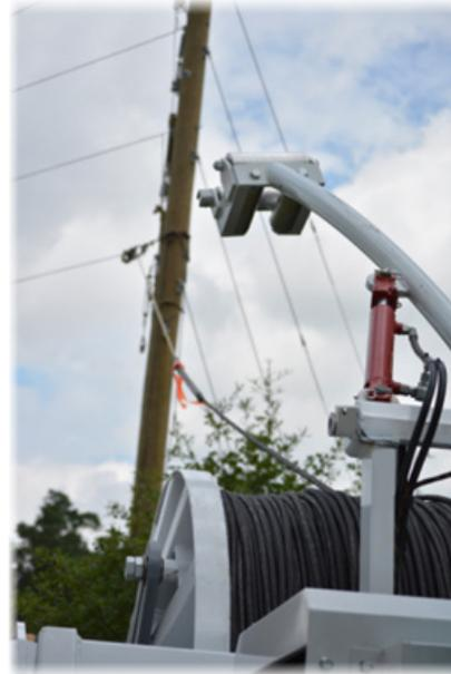
**NOTE:** In some situations, (i.e., due to rough terrain), it may not be possible to achieve these safe distances from the lead block. In these situations, operators should try and achieve as much distance as possible from the lead block and be aware of the increased down forces during operations.
