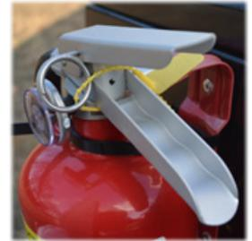
**NOTE:** If the safety seal is missing or is broken, extinguisher may have been tampered with or may have already been used- indicating the need for re-inspection/replacement.
