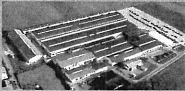
Plant I, Gremsdorf, Germany
